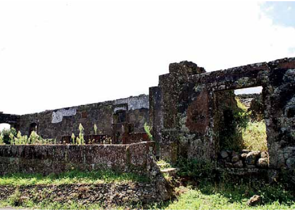
Figure 45. The “Solar dos Tiagos” in ruins, Topo
